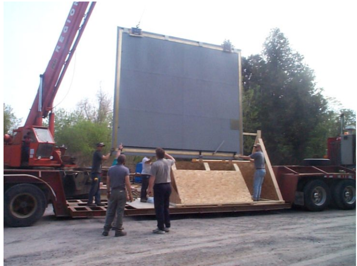
A 12' x 14' Single leaf QuietDoor being loaded onto a low bed trailer for delivery
